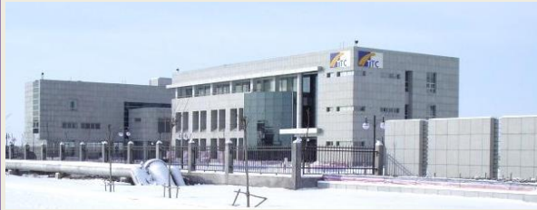
Tianjin plant (Est. since Sept. 2005)
