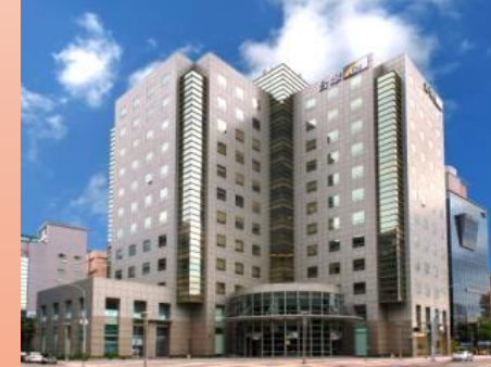
Taipei head office Neihu Technology Park
