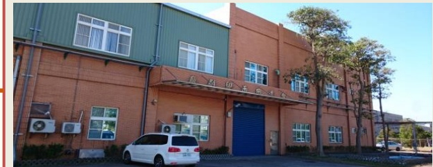
Glasswool plant (Est. since Mar., 1991) Cubic plant (Est. since Jun., 1987)
